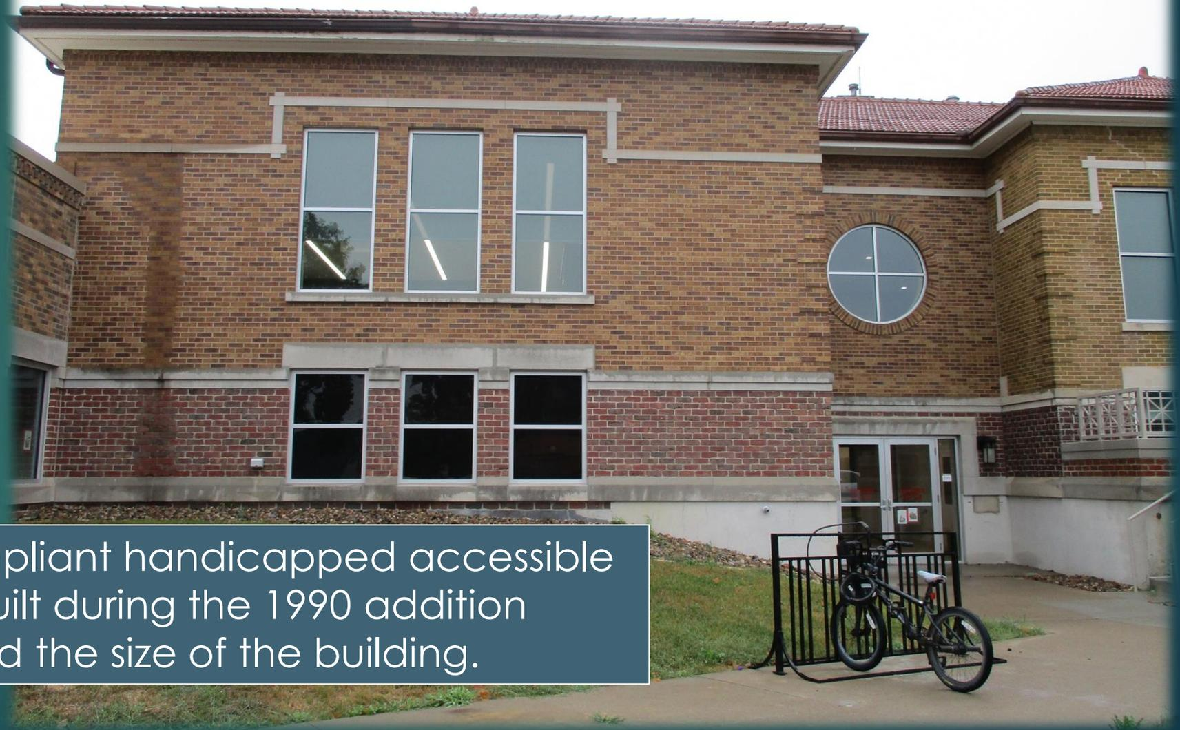
This sloped ADA compliant handicapped accessible entrance was built during the 1990 addition which doubled the size of the building.
